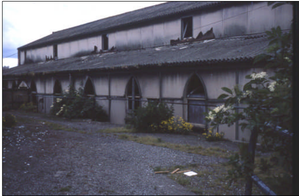
The Irwell Street church awaits the bulldozers. The Busway now passes through the site. There is not a trace of the first two churches dedicated to St. Edward.
